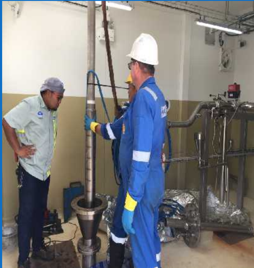
Re-install pump and transducer
